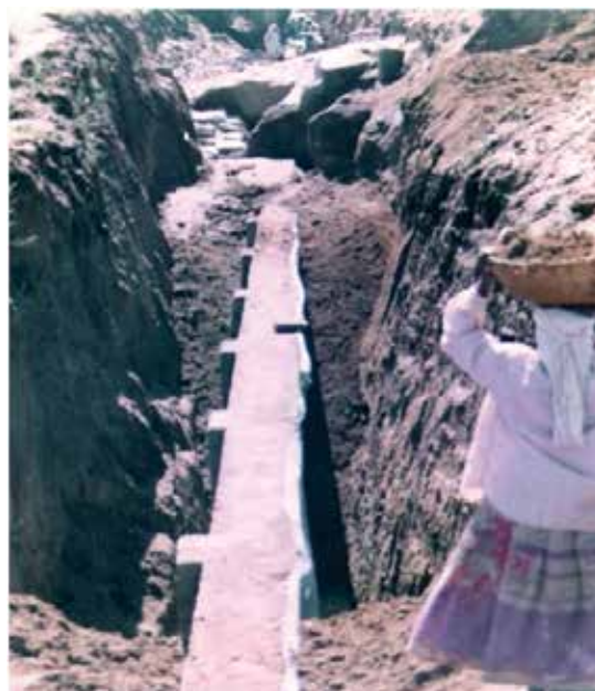
Figure 11. Design of a sub-surface dike for management of the base flow to create storage and recharge to groundwater, Palghat District, Kerala.
