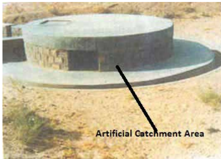
Figure 2. A tanka or underground storage cement structure with an artificial catchment area, a 10 th century structure.
