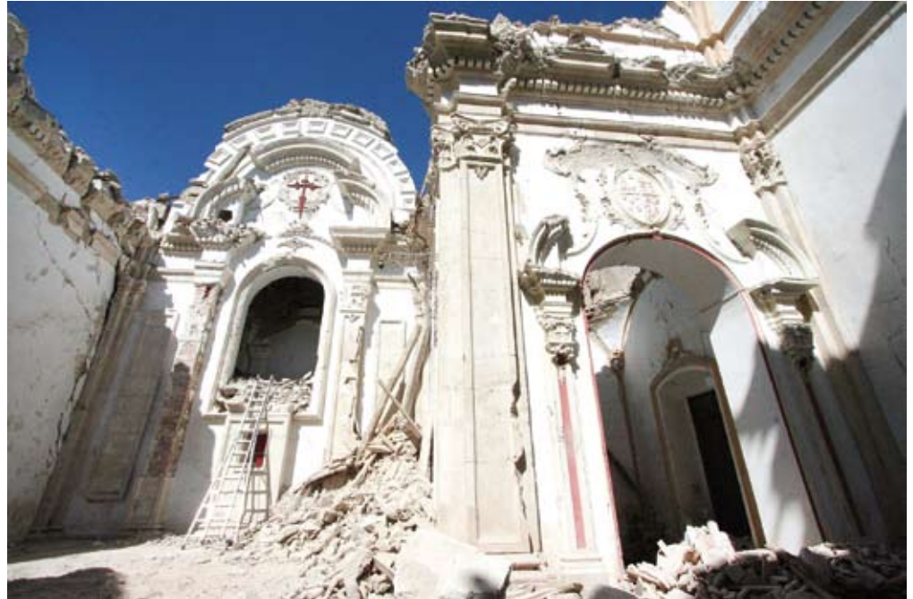
Figura 23. Retirada de material del desplome del crucero de la Iglesia de Santiago con supervisión arqueológica. Figure 23. Removal of debris from the collapsed transept of the church of Santiago under archaeological supervision.
