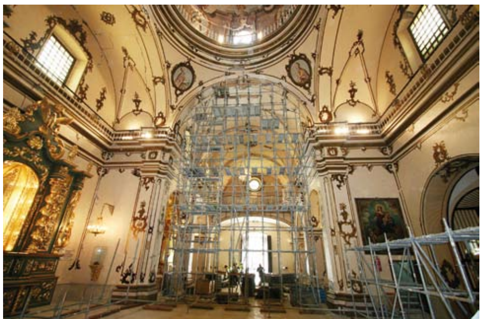
Figure 18. Propping up of the arches over the transept of the El Rosario chapel.
