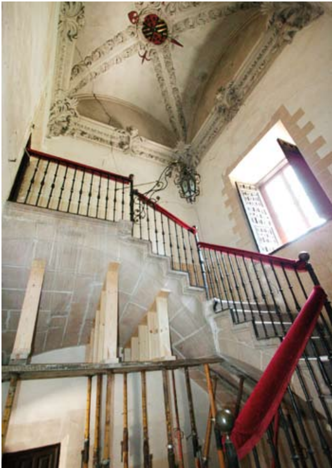
Figura 24. Apeo de la escalera principal del Palacio Guevara. Figure 24. Propping up of the main staircase of the Guevara palace.
