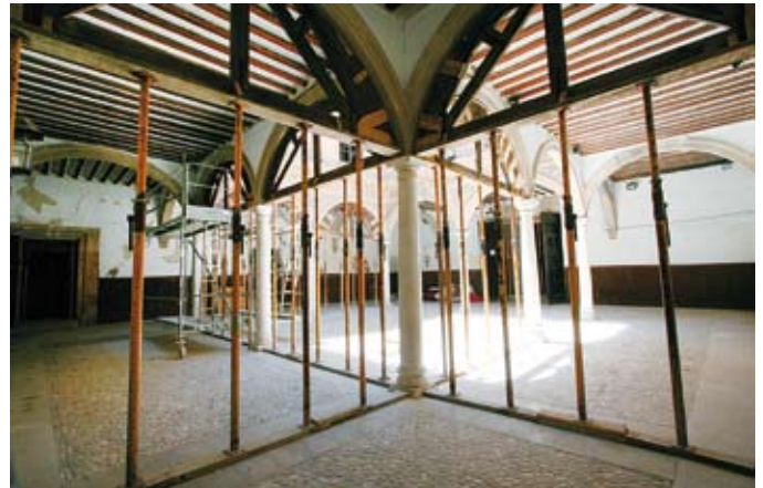
Figura 25. Apeo de los arcos del patio y forjados de planta primera del Palacio Guevara. Figure 25. Propping up of the arches of the courtyard and first-floor iron beams at the Guevara palace.
