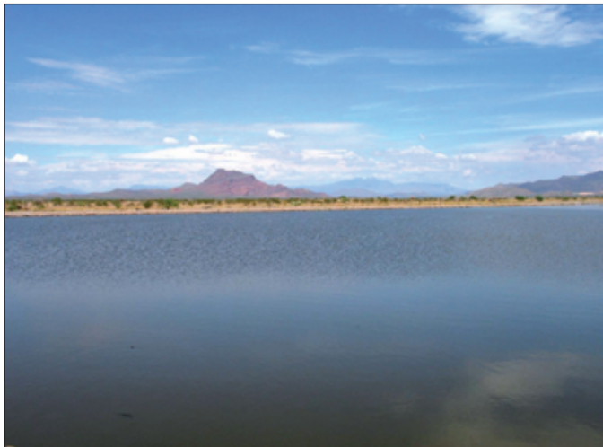
Figure 2. Recharge basin of the Granite Reef Underground Storage Project. This basin has a surface area of 25 hectares and an infiltration rate of one meter per day
